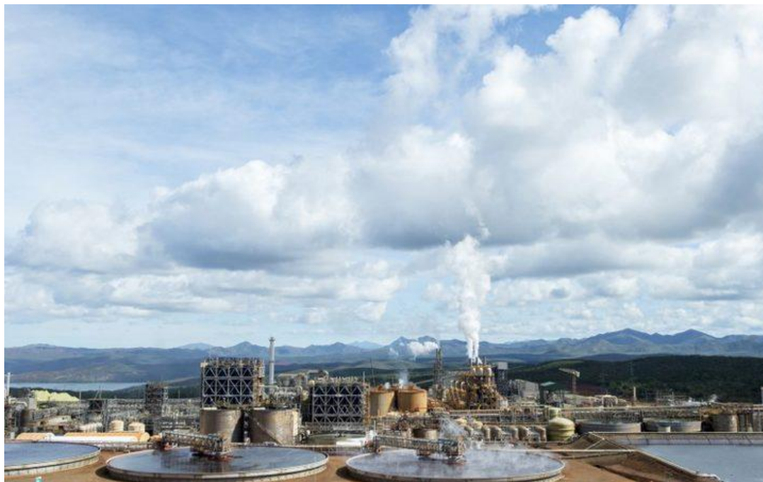
A photo taken on May 27, 2015 shows Brazilian Vale's nickel processing plant of Goro in southern New Caledonia. Photo: AFP PHOTO / FRED PAYET
