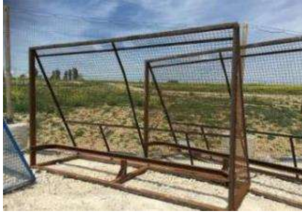
Figure 5: Pose des cages anti-envol
